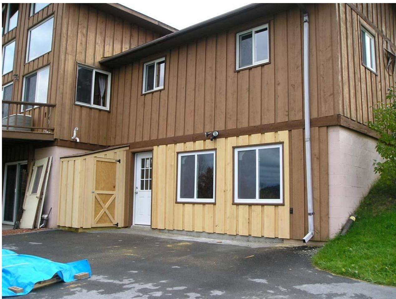
The outside of the old garage was also re-done. Two new windows and a door added, plus a small shed in the corner. The siding was specially cut to match the old house siding.
